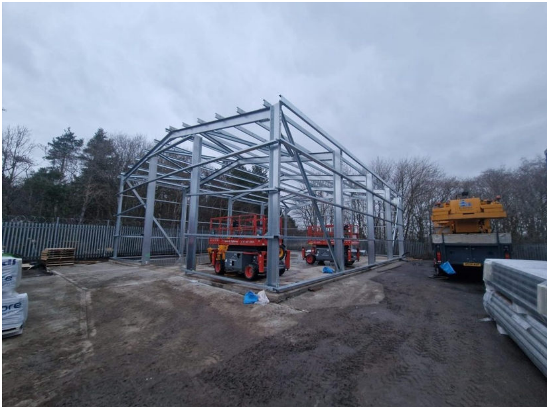
GALVANISED PORTAL FRAME UNDER CONSTRUCTION
