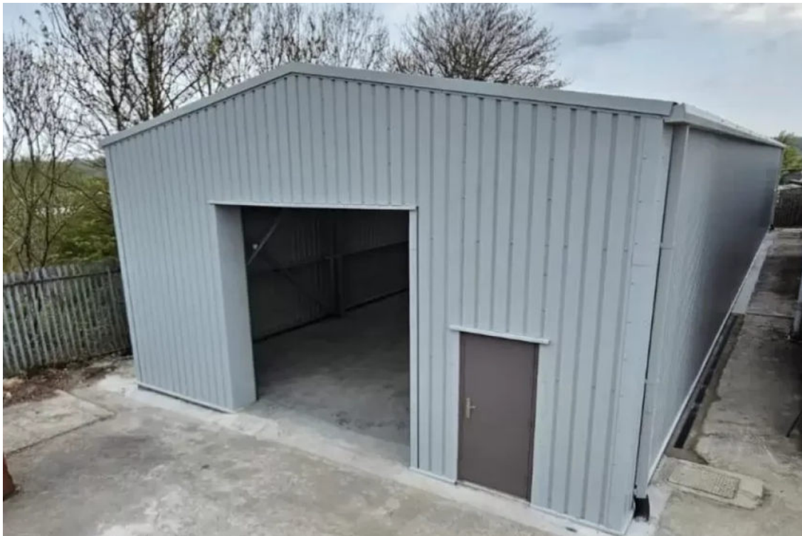
JOHN CLARK VALVES / STEEL BUILDING EXTENSION
