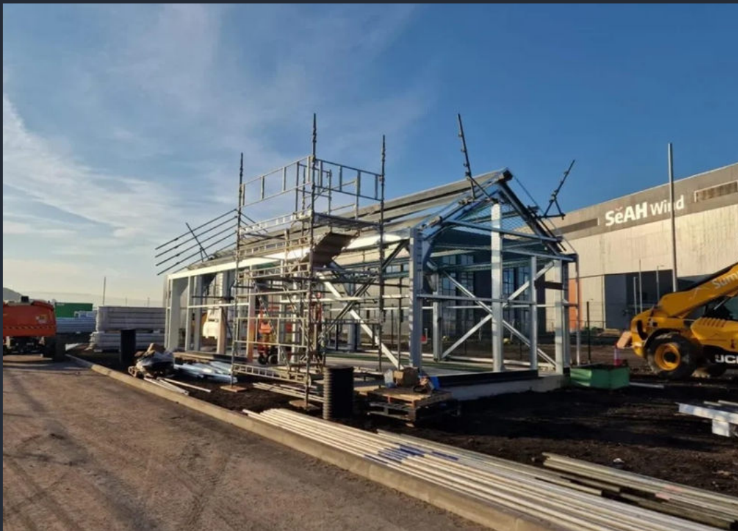
TEESWORKS / FRAME ERECTION & EDGE PROTECTION
